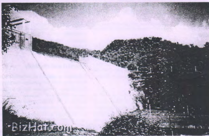
Figure-2 Sothuparai Dam
